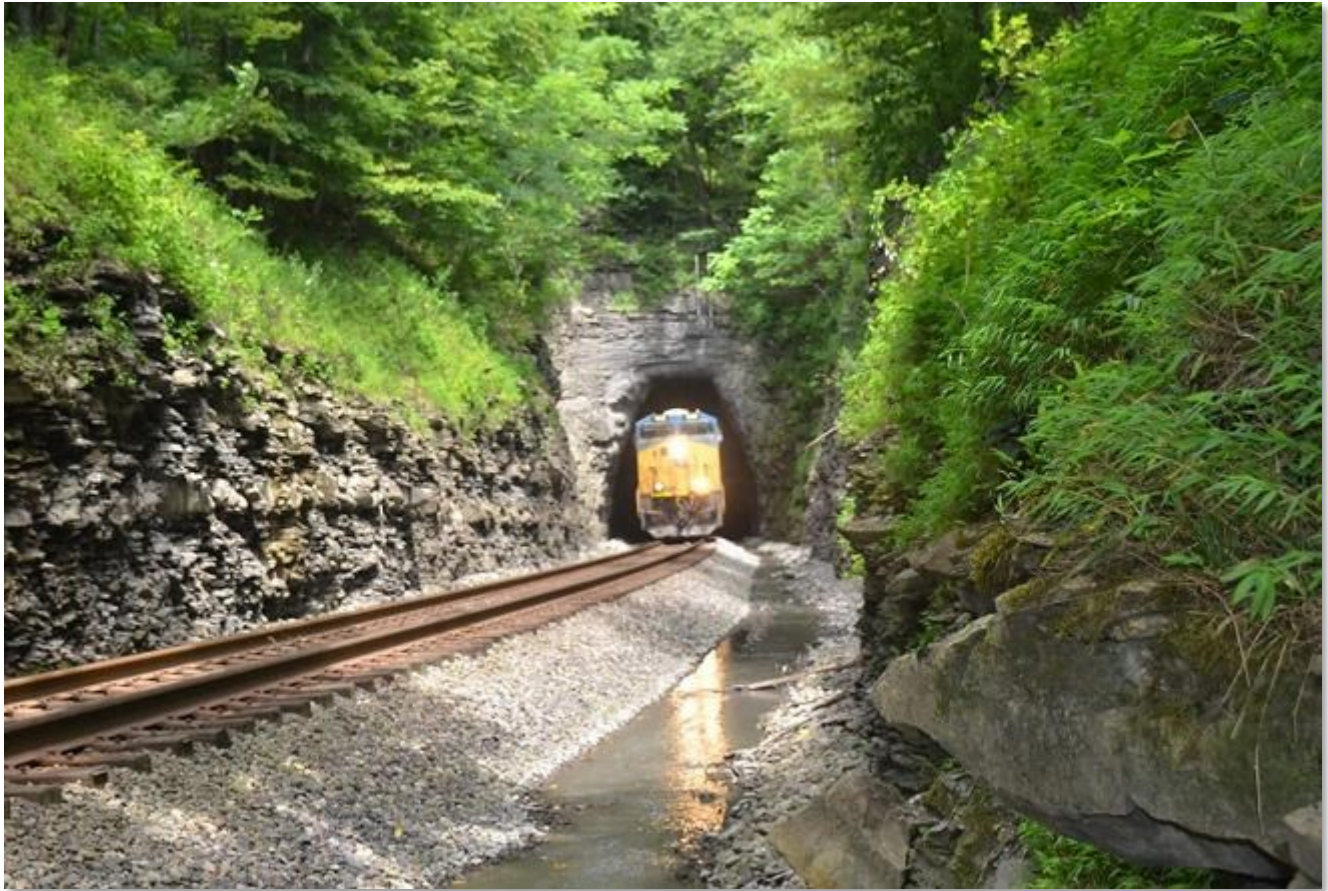
Second Place, July 2019, West Kentucky NRHS Photo Contest - CSX locomotive # 958 pulls an intermodal south on the Henderson Subdivision after emerging from the south portal of Ridgetop Tunnel, north of Baker Station crossing in Ridgetop Tennessee on May 30, 2019. - Photo by Bill Farrell.
